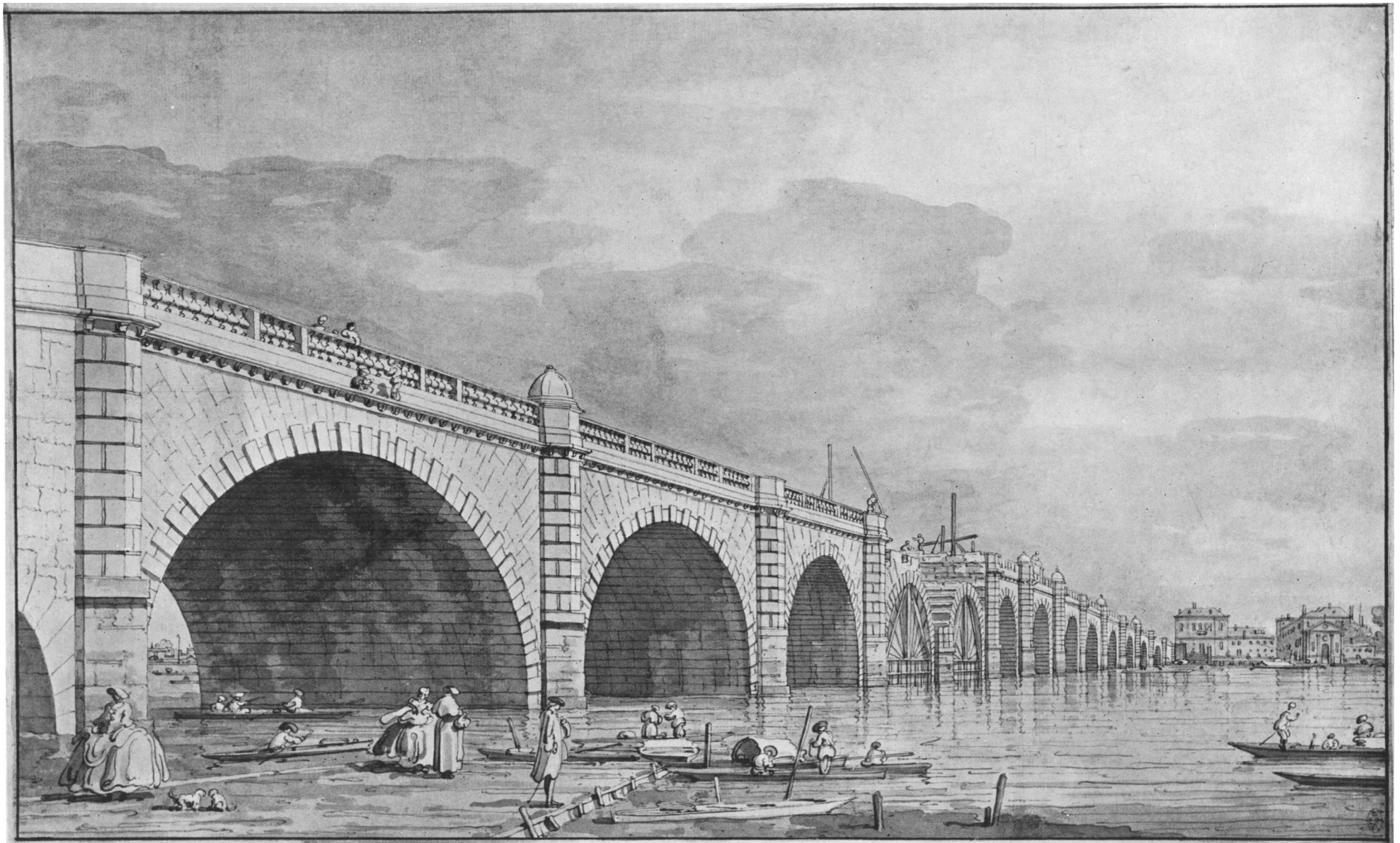
76. LONDON: WESTMINSTER BRIDGE UNDER CONSTRUCTION (Cat. No. 118)
